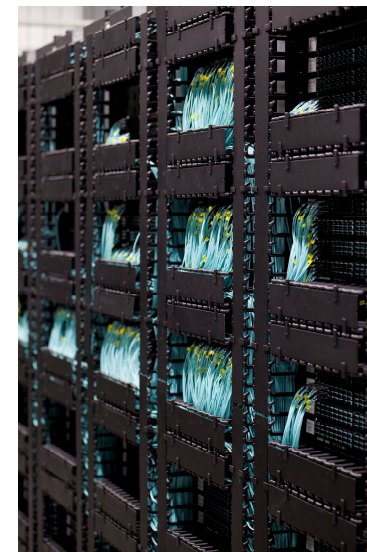
Rosenberger OSI Cable Management System in a Data Center's patch distributor and equipment rack
